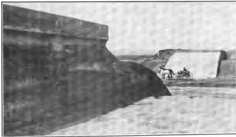
FIG. 153.—Siphon Crossing under Rawhide Creek, Interstate Canal, Nebraska-Wyoming.
